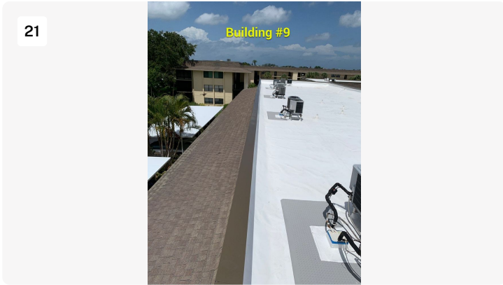
Building #9 facing west
