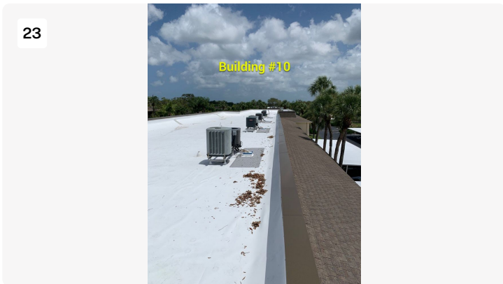
Building #10 facing north
