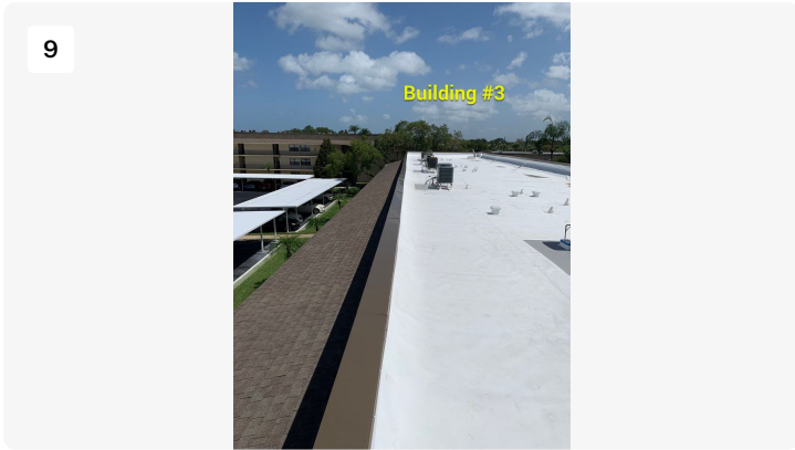
Building #3 facing north
