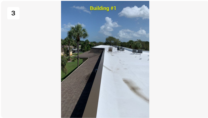
Building #1 facing north
