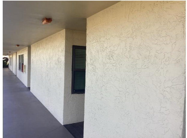
Stucco wall finishes at breezeway
