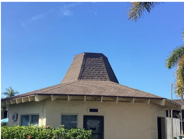
Roof at maintenance building
