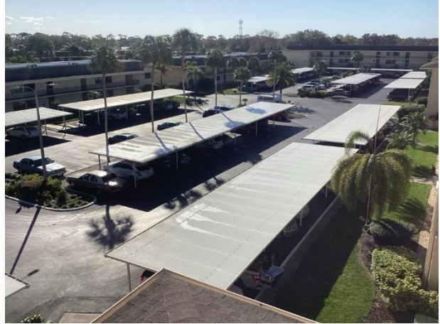
Carport roofs overview
