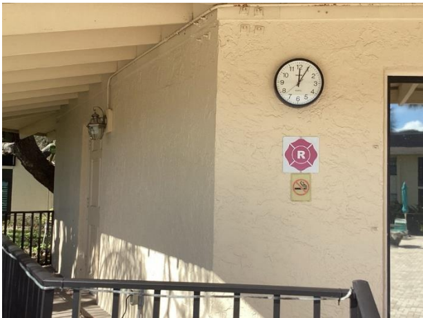
Stucco wall finishes at pool hall
