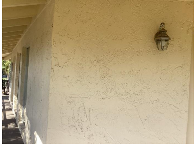
Stucco wall finishes at clubhouse
