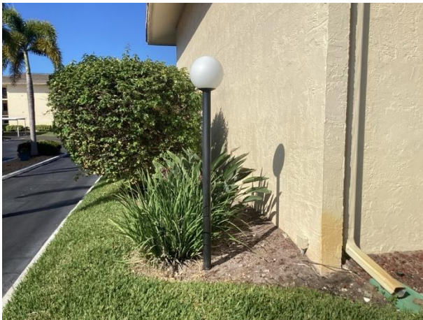
Light pole and fixture
