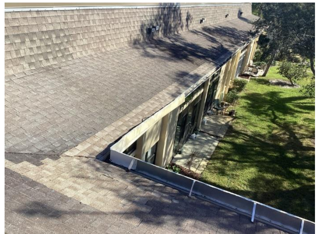
Residential roof with previous repair along edge
