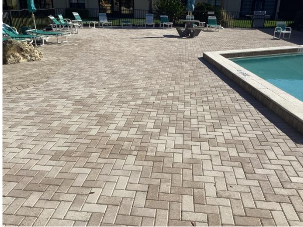
Paver pool deck overview
