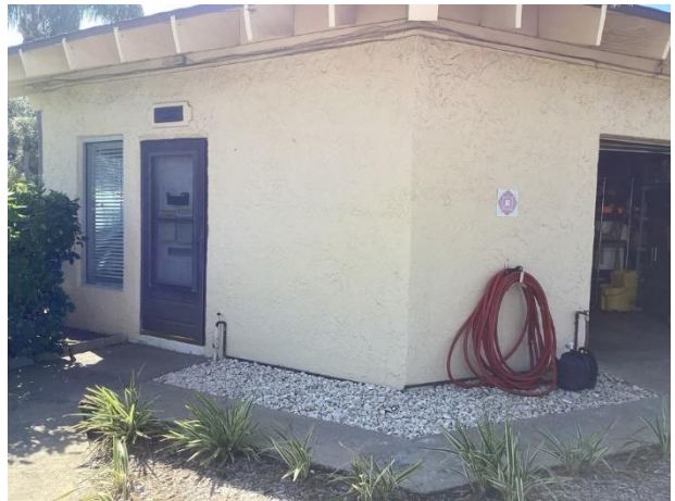
Stucco wall finishes at maintenance building
