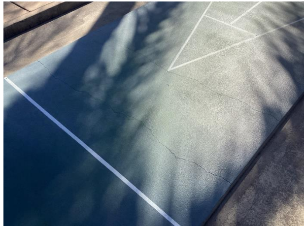
Shuffleboard cracks
