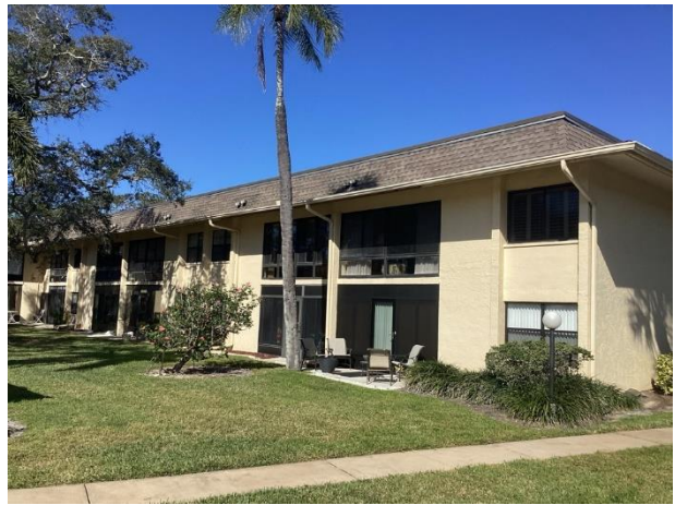
Rear elevation of two-story building
