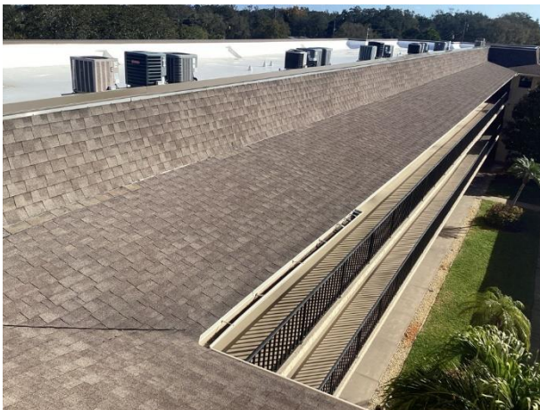
Asphalt shingle roof at residential building
