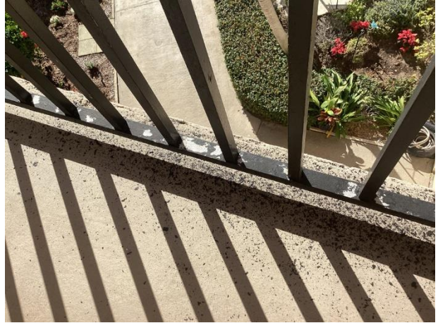
Aluminum railings being repaired
