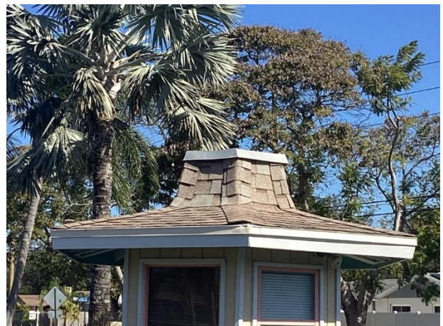
Roof at guardhouse
