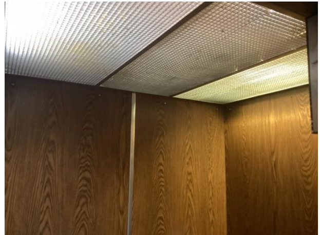
Elevator cab finishes
