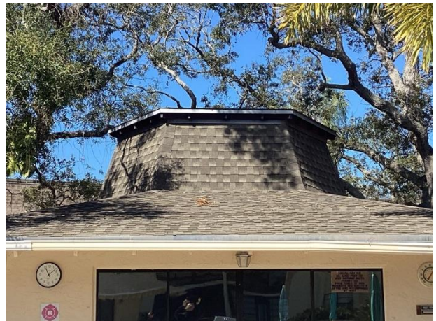
Roof at pool hall
