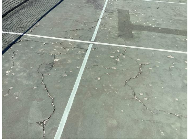
Surface cracks
