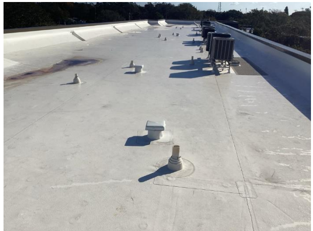
Thermoplastic roof overview
