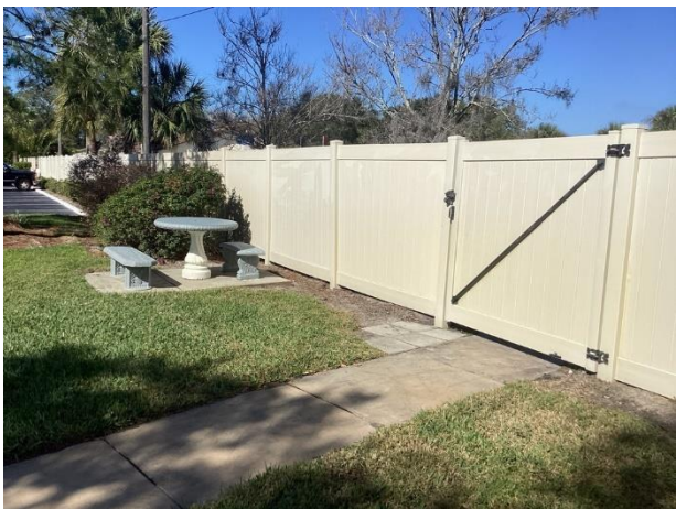
Vinyl fence at north perimeter
