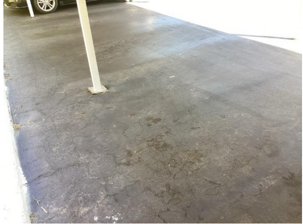
Pavement under carport
