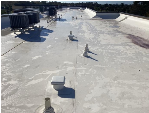
Thermoplastic roof overview
