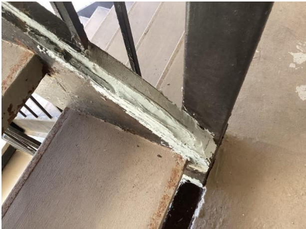
Metal staircase being repaired
