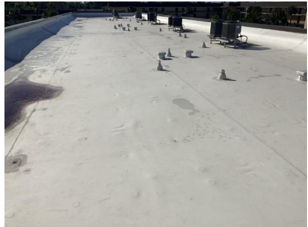
Flat roof overview
